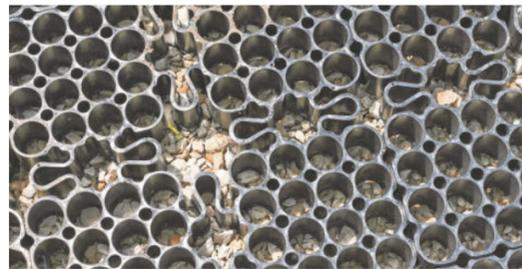
The Pella Grid System uses cylinders made out of recycled plastic filled with pea rock to create an even surface area for walking and driving. The system absorbs water instead of creating runoff.
